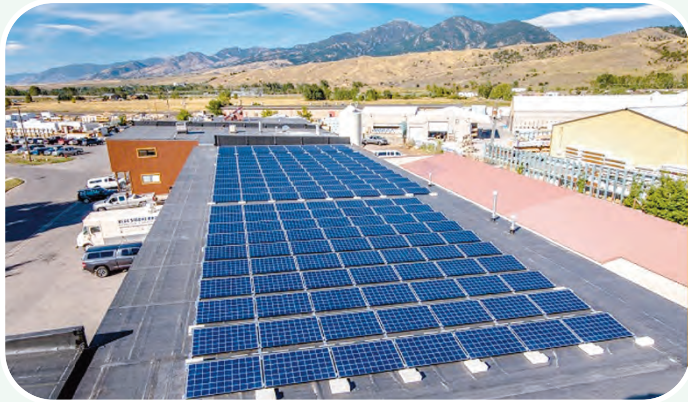
Bozeman Brewing Company roof - www.harvestsolarmt.com
