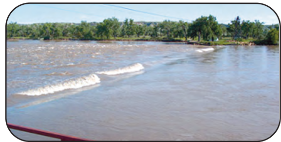
Lower Yellowstone Diversion Dam, Mont.
